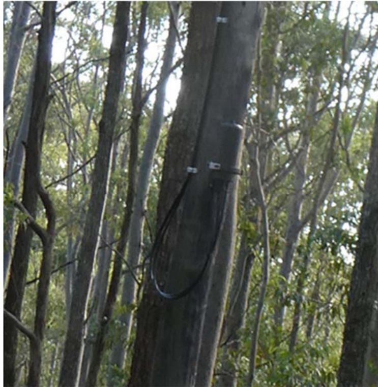
Figure 3 – Typical 10/0.64 pole mounted joint on aerial cable.
