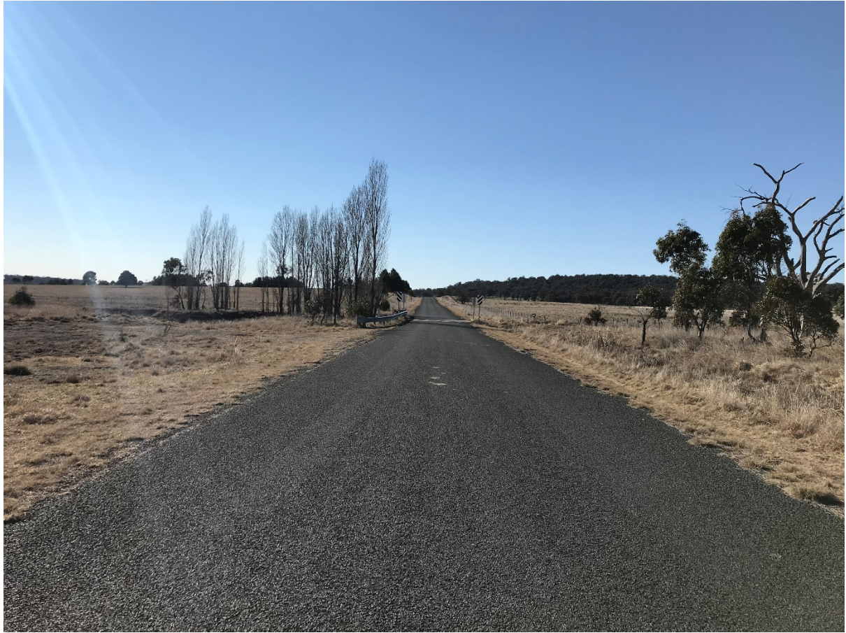
Photograph A.1: Big Ridge Road within Segment 2, approximately 2 km from intersection with Barleyfields Road, looking east
