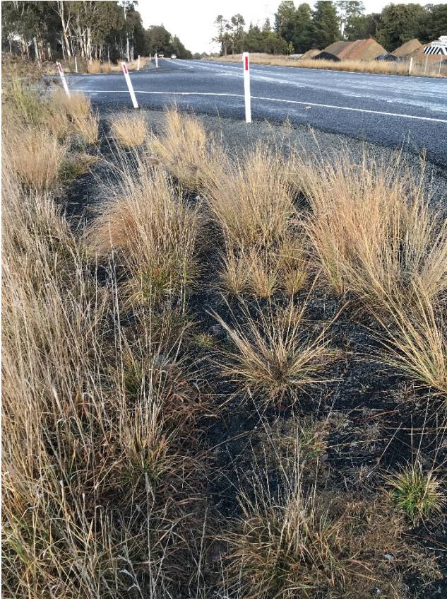
Plate 4.1 Survey transect 1 - view south-west showing disturbance from initial construction of the New England Highway
