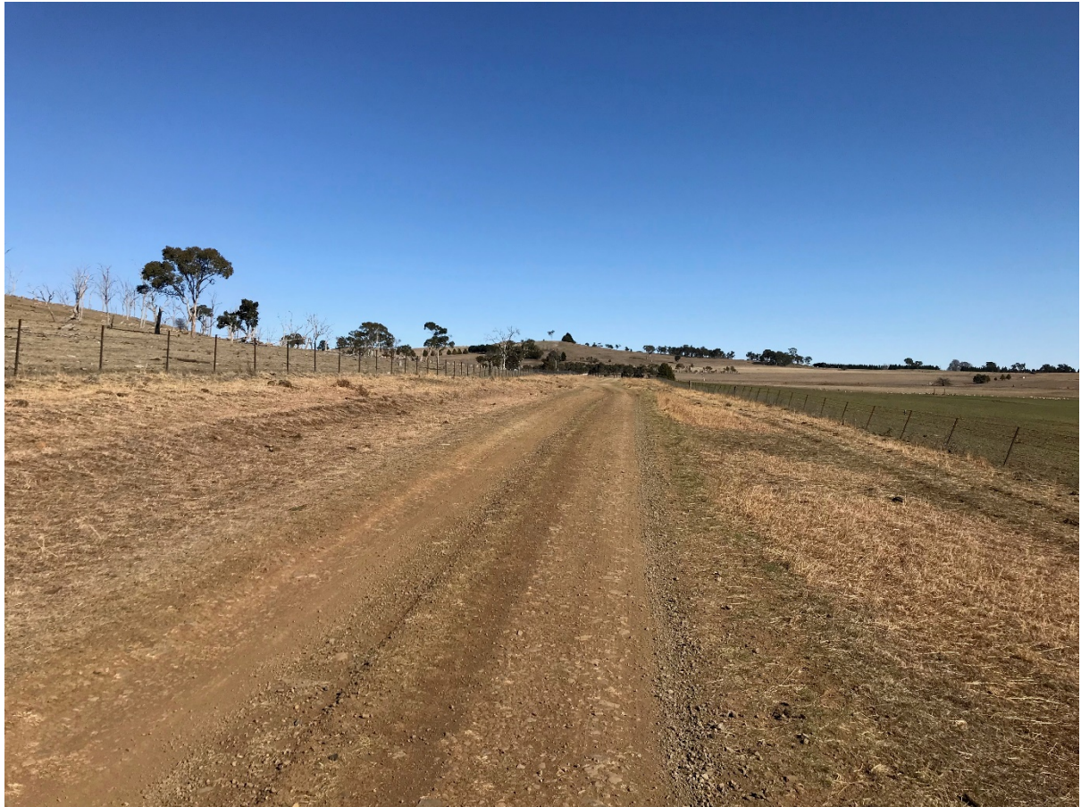
Photograph A.4: Big Ridge Road within Segment 4, approximately 8 km from intersection with Barleyfields Road, looking west
