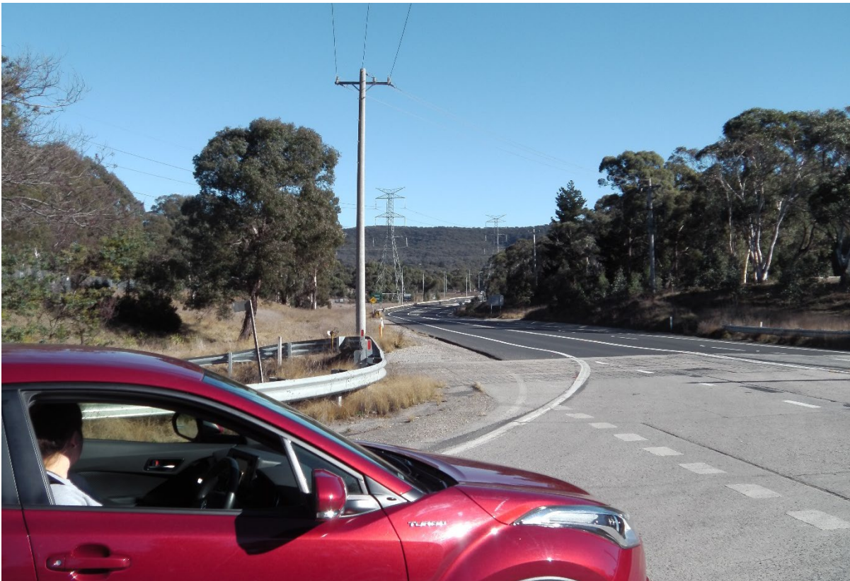
Photograph C.1 Visibility at intersection looking west from the haul road towards Wolgan Road (23 July 2019)
