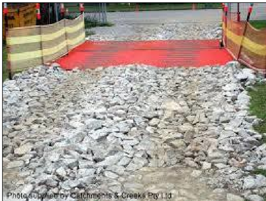
Figure 5.2 Gravel haul road to be installed at Marine Berth and Emplacement Cell Construction Sites
