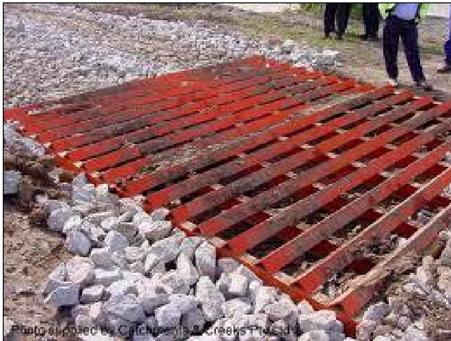
Figure 5.1 Rumble grid to be installed at Marine Berth and Emplacement Cell Construction Sites
