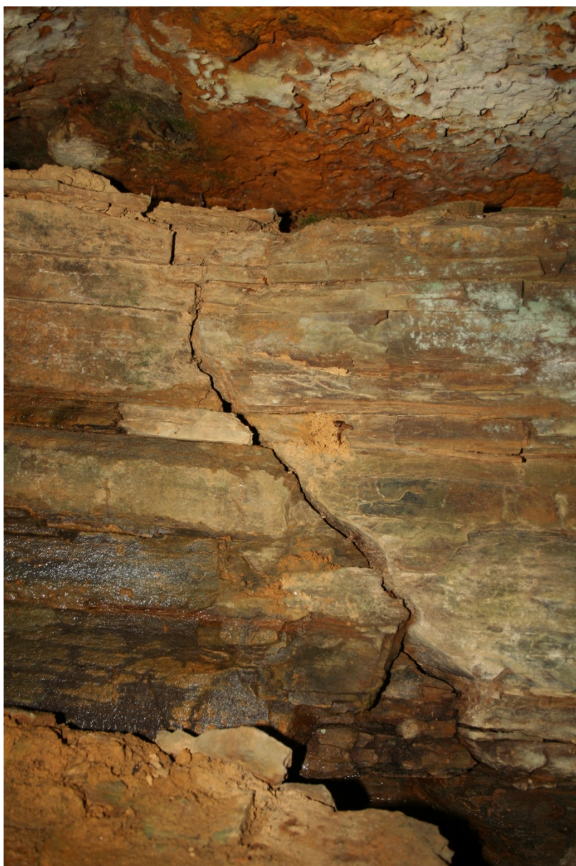
Bulli Mine Shaft 20 – interior of shelter showing cracking and water seepage, facing north-west
