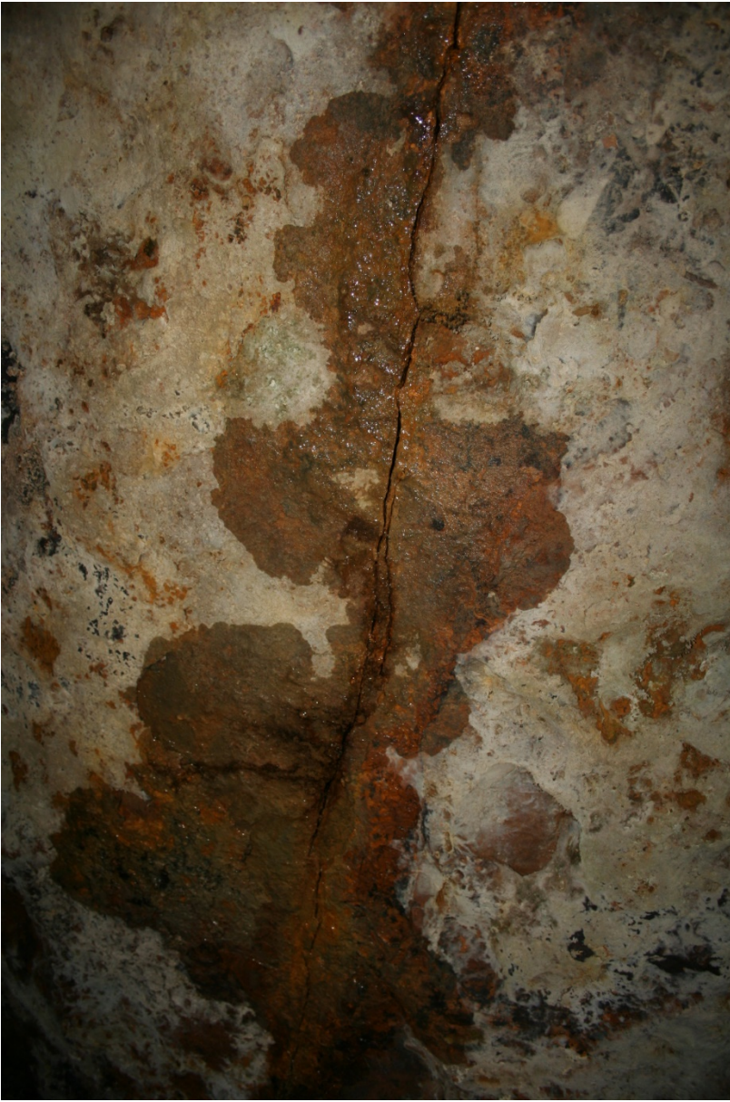
Bulli Mine Shaft 20 – interior of shelter showing cracking and water seepage
