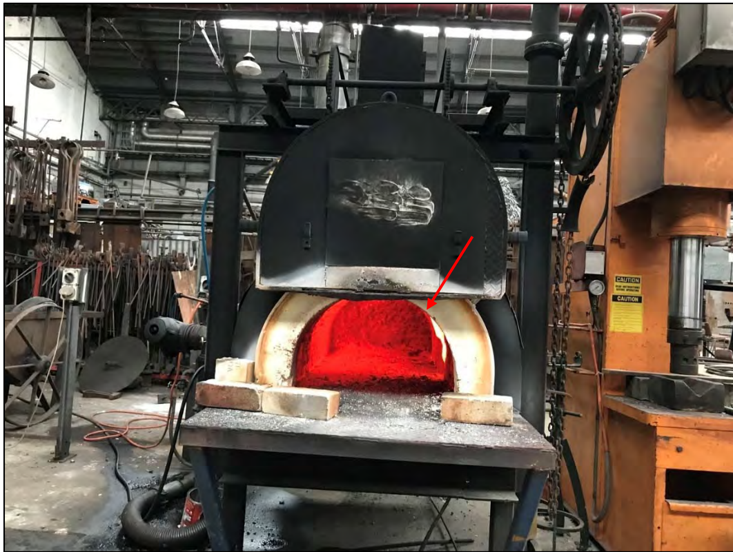
Photograph 5: The Big Major Oil Furnace reaches efficient burn operation after 20 – 30 minutes as the refractory heats to optimum temperature.
