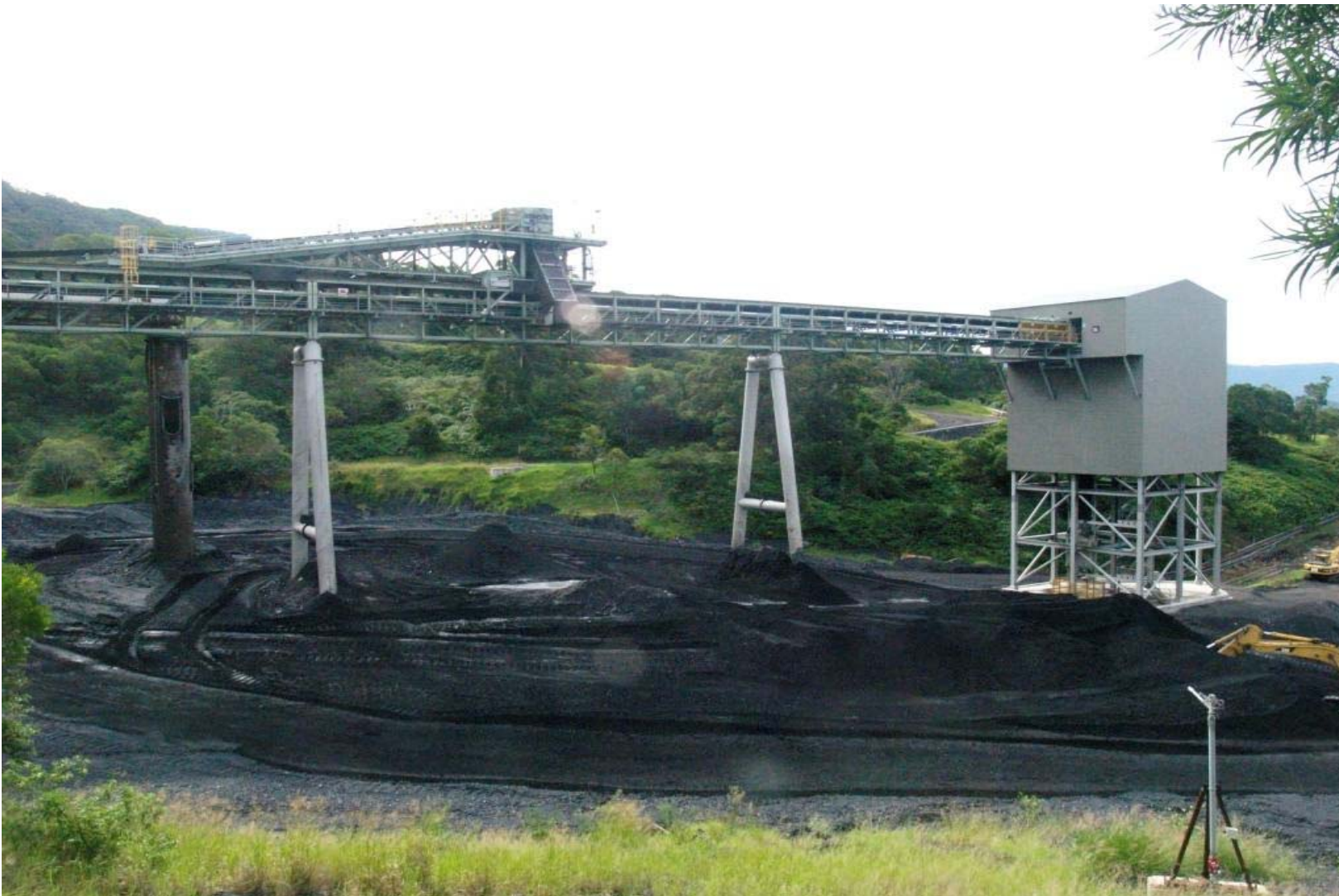
Figure 3.2: View of stockpile conveyor, tripper and conveyor drive house
