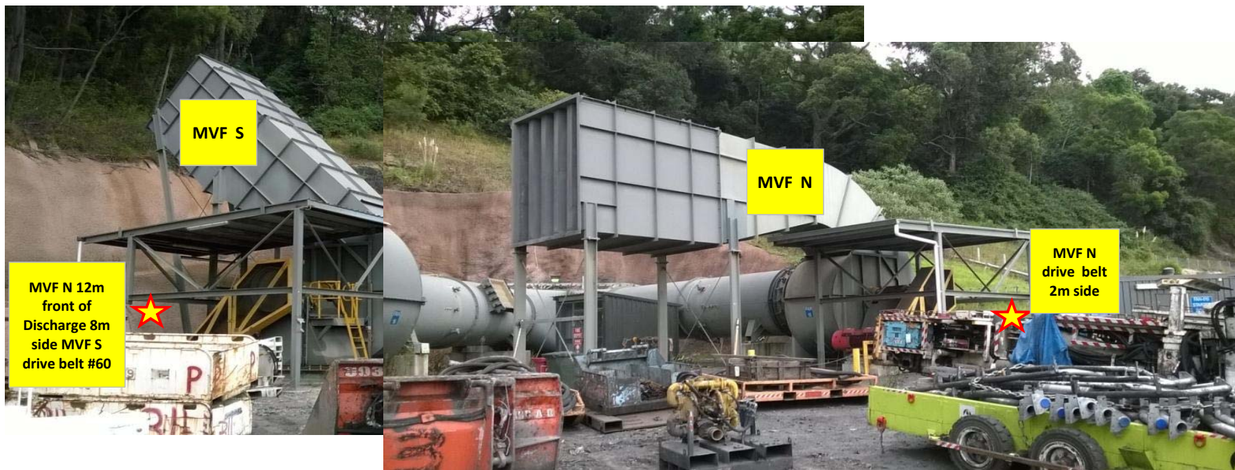
Figure 3.5: View of Mine Ventilation Fans and measurement locations
