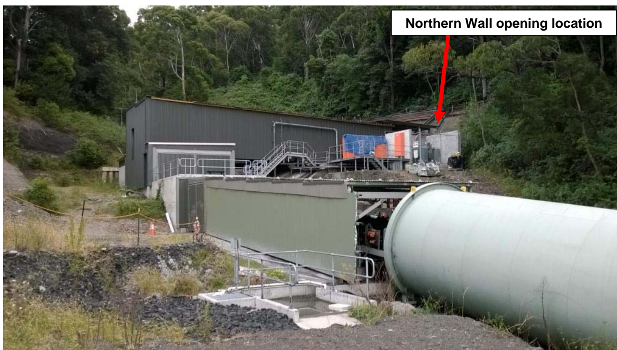
Figure 6.21: View of the Sizer building, connection to the conveyor gantry tube and area of the northern wall opening at the Portal.
