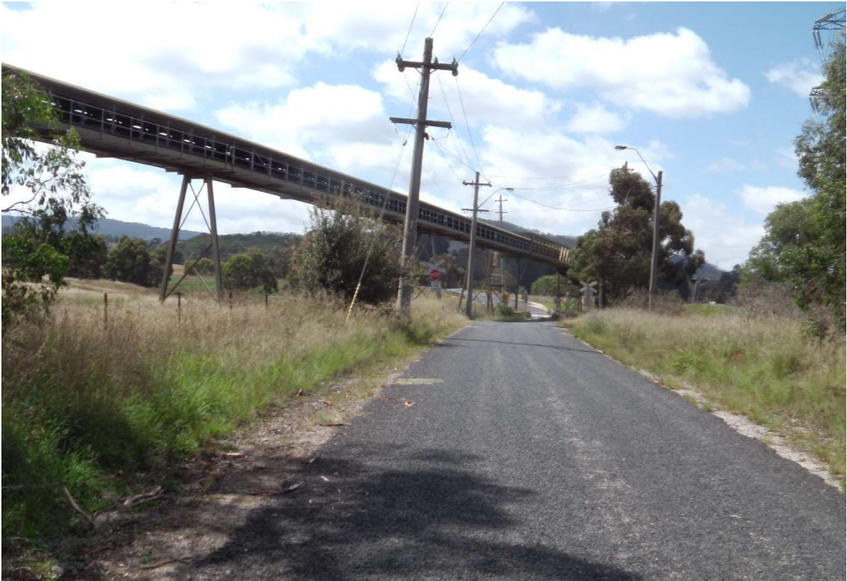
Brays Lane at proposed access looking east
