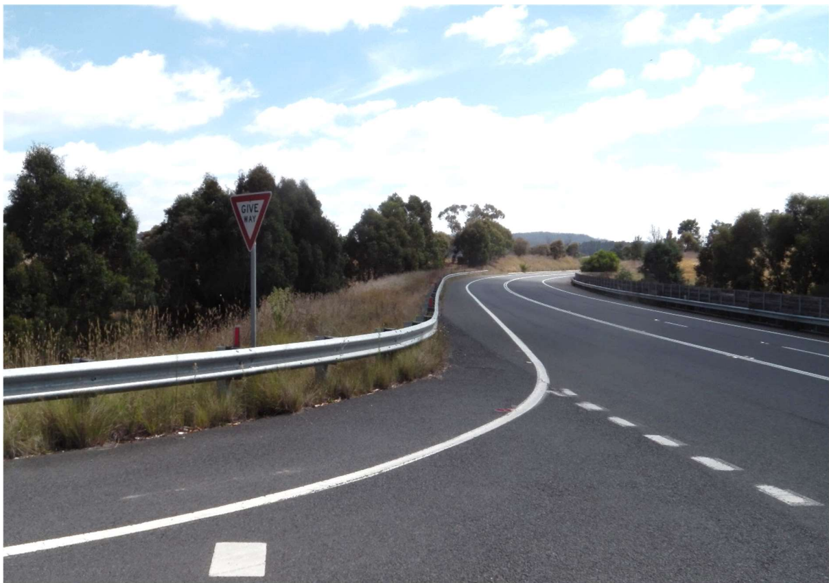
Castlereagh Highway at Brays Lane looking left
