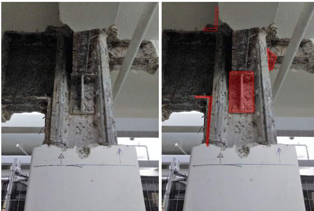
Figure 5 Exposed steel column connection at TC6 (left), with angle support brackets highlighted (right)
