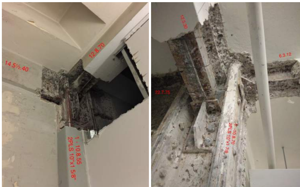
Figure 3 TC4 (left) TC6 (right) column/beam locations after removal of concrete encasement
