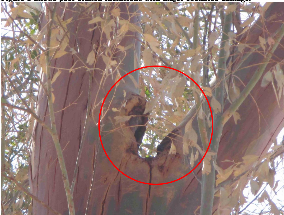
Figure 6 Shows a close up of a poor branch union.
