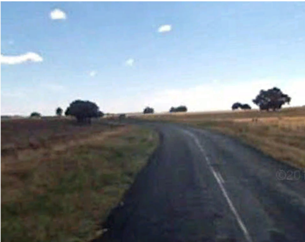
Figure 7. Google Earth Snapshot (Northbound Carriageway)
