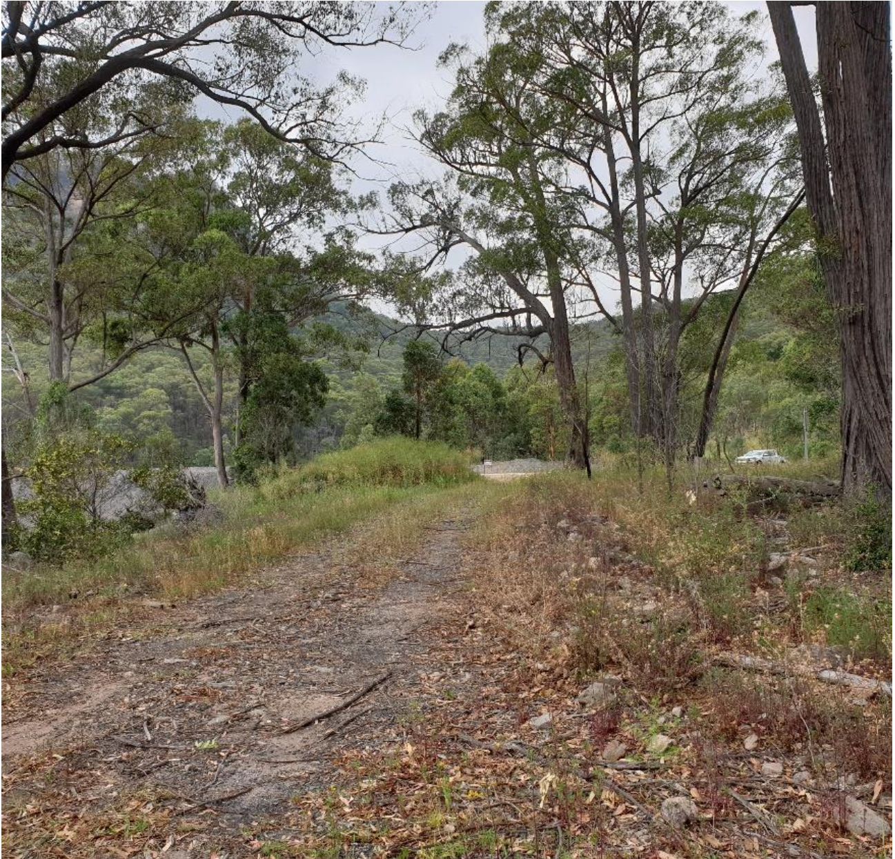
Plate 1 Area of road to be widened in PCT 1088
