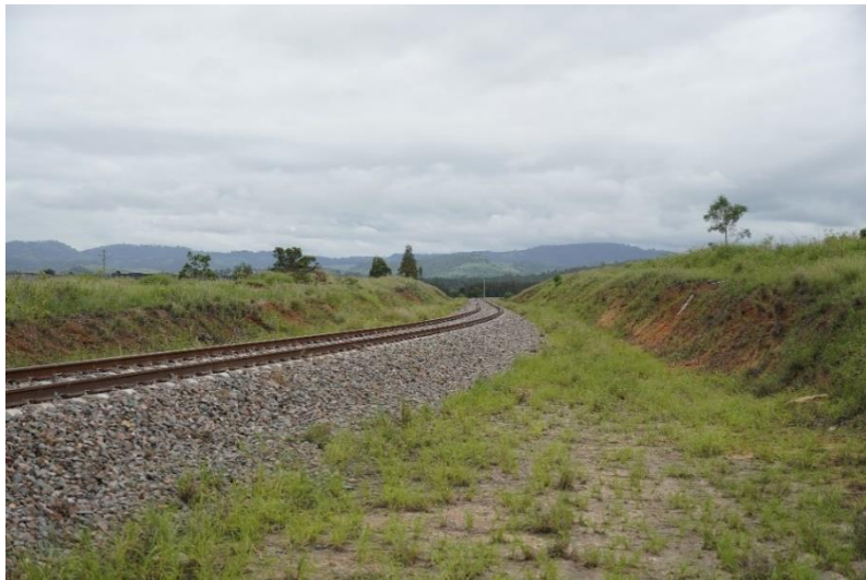
Figure 4-13 Railway cutting – Cut 5
