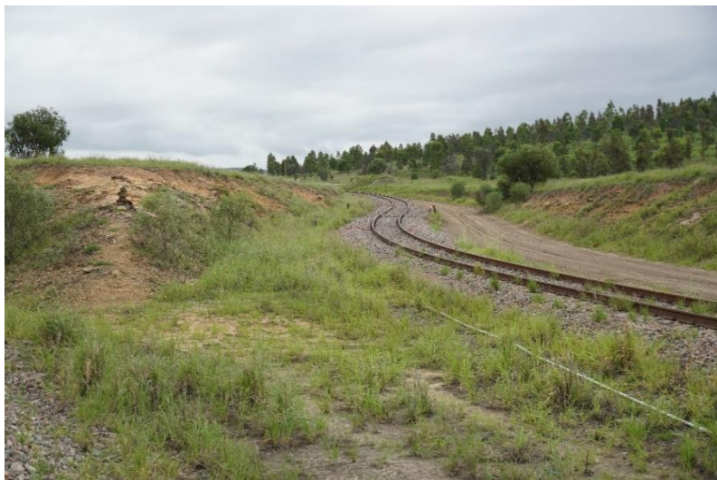
Figure 4-14 Railway cutting – Cut 6
