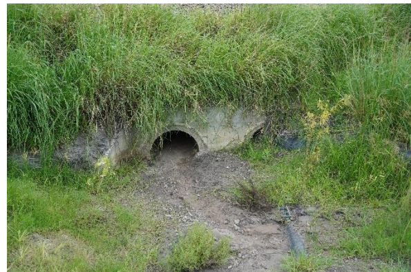
Figure 4-17 Concrete culverts C4 (left-hand side) and C5 (right-hand side)
