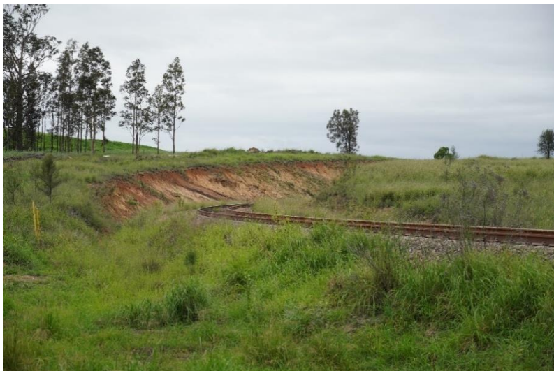
Figure 4-11 Railway cutting – Cut 3
