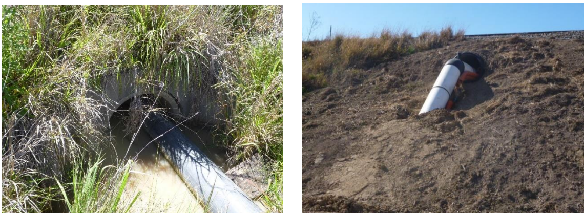
Figure 4-15 Concrete culverts C1 (left-hand side) and C2 (right-hand side)
