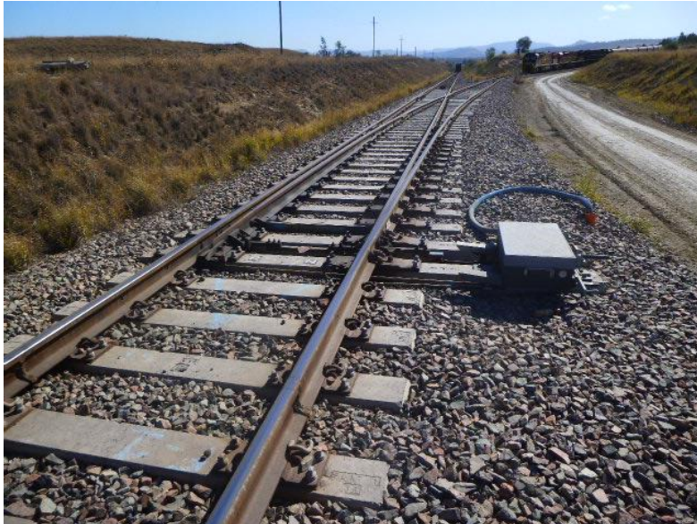
Figure 4-5 Railway switch at southern end of Railway loop
