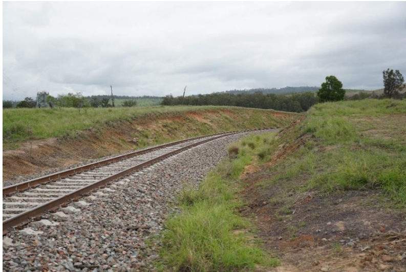
Figure 4-12 Railway cutting – Cut 4
