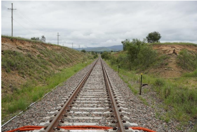
Figure 4-9 Railway cutting – Cut 1
