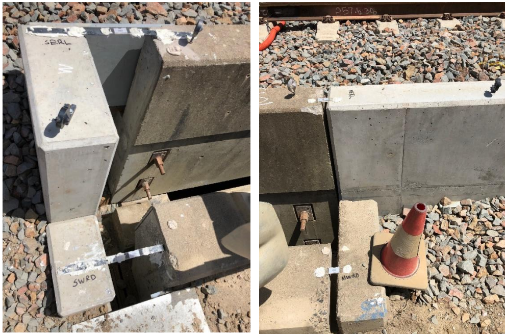
Existing 3D monitoring points and tell-tales on the Bridges
