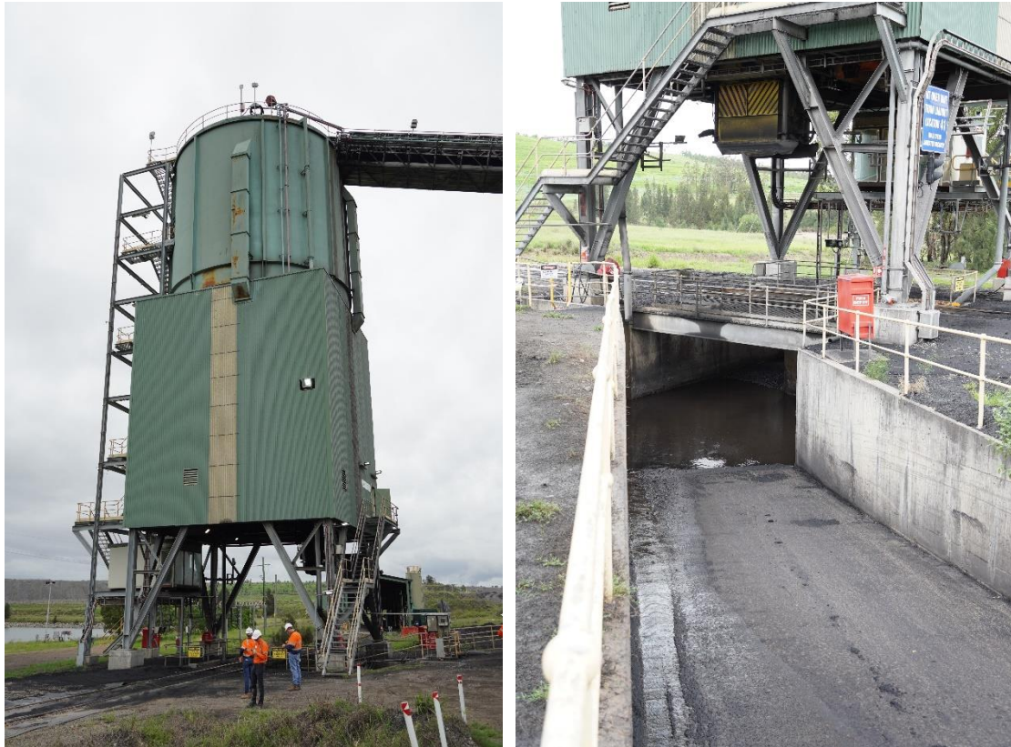
Figure 4-19 Coal loading bin and inground pit
