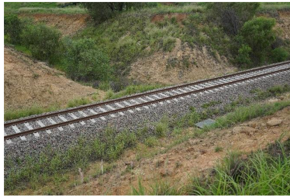
Figure 4-16 Concrete culvert C3
