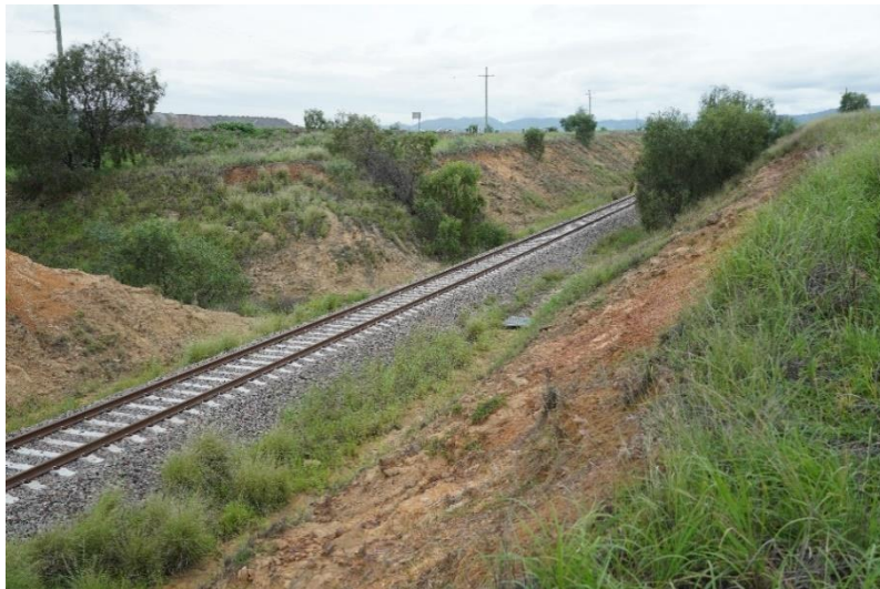
Figure 4-10 Railway cutting – Cut 2
