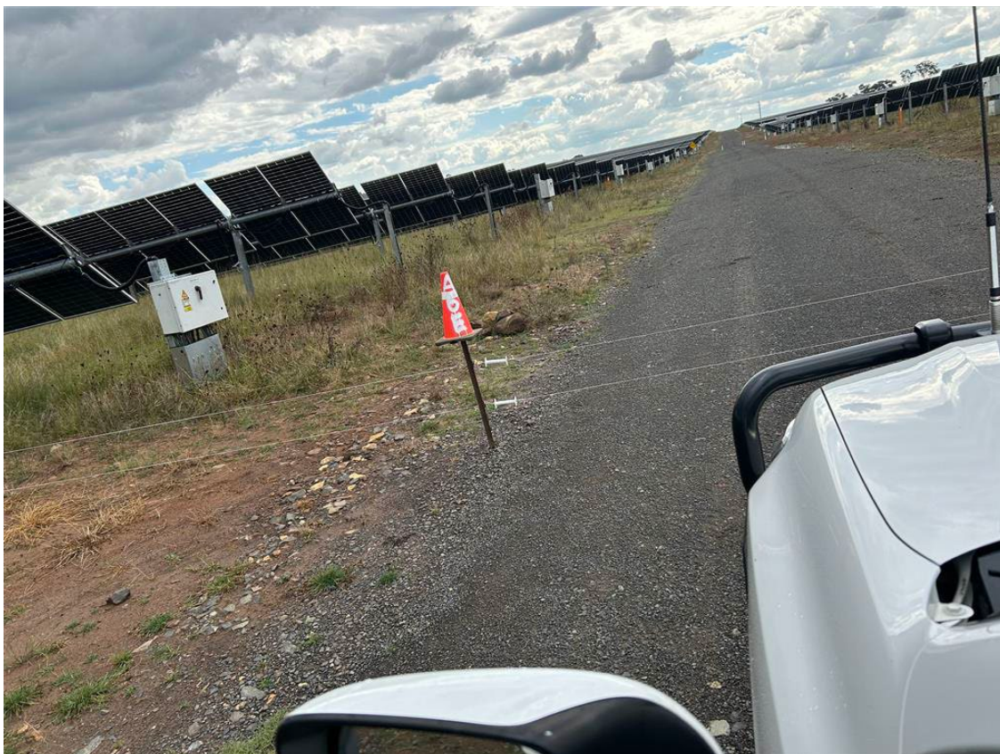
Figure 7 – Temporary electric fence between solar arrays.
