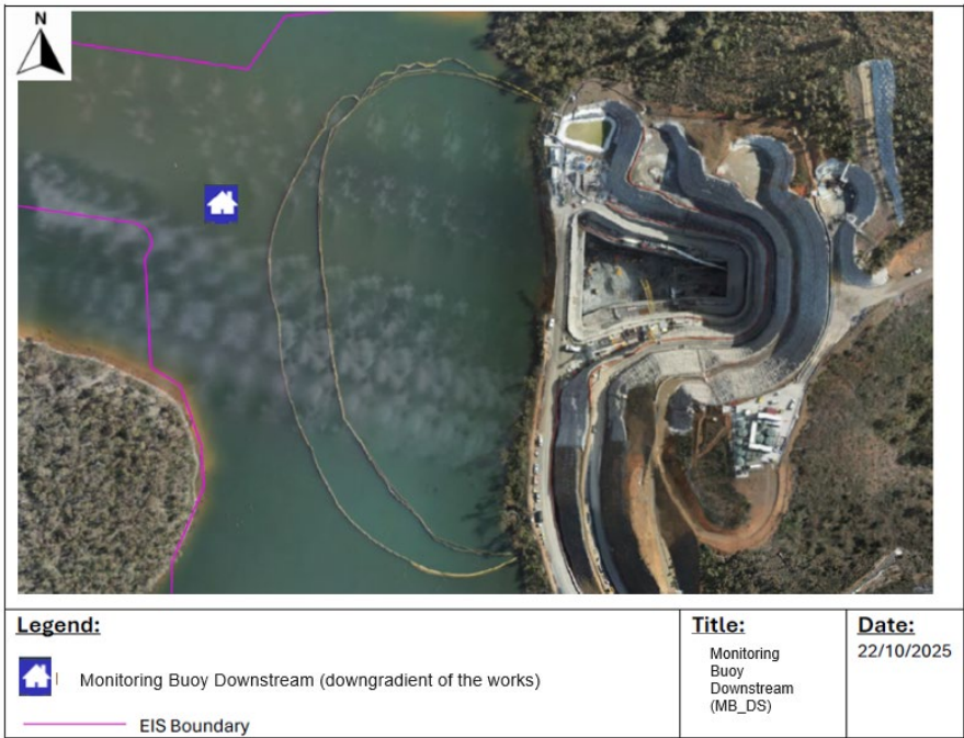
Figure 7-3 EPL11 - Downstream Monitoring Buoy Locations
