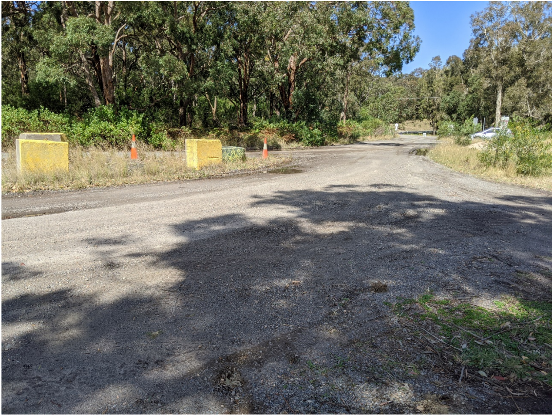
Photo 8: Site entry/exit onto Coxs Lane
