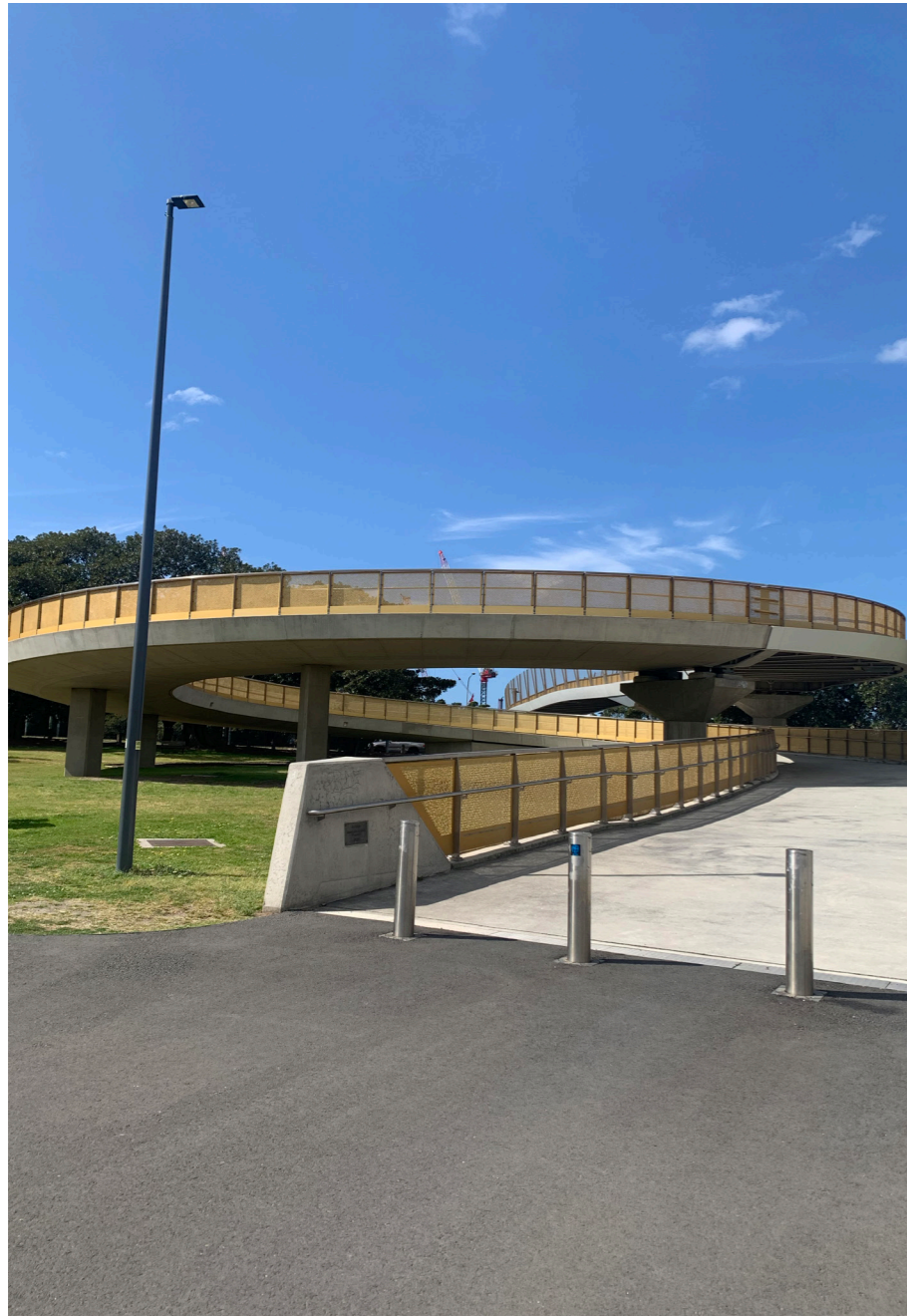
The site is approximately 2km from Central Station, making it a comfortable 25 minute walk for large crowds attending events at Moore Park. The precinct is accessible from Central via Devonshire Street and the Albert 'Tibby' Cotter Walkway.
