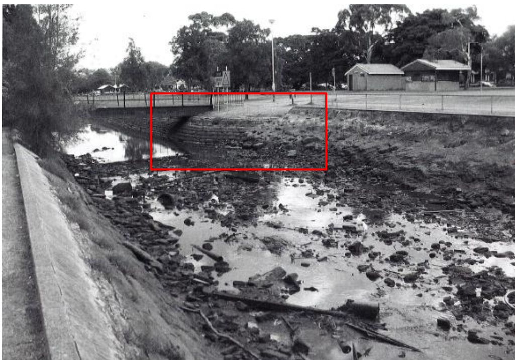
Figure 9. Sediment and base of Hawthorne Canal and merging point of old and new walls, 2004. (Source: Mark Sabolch). 5
