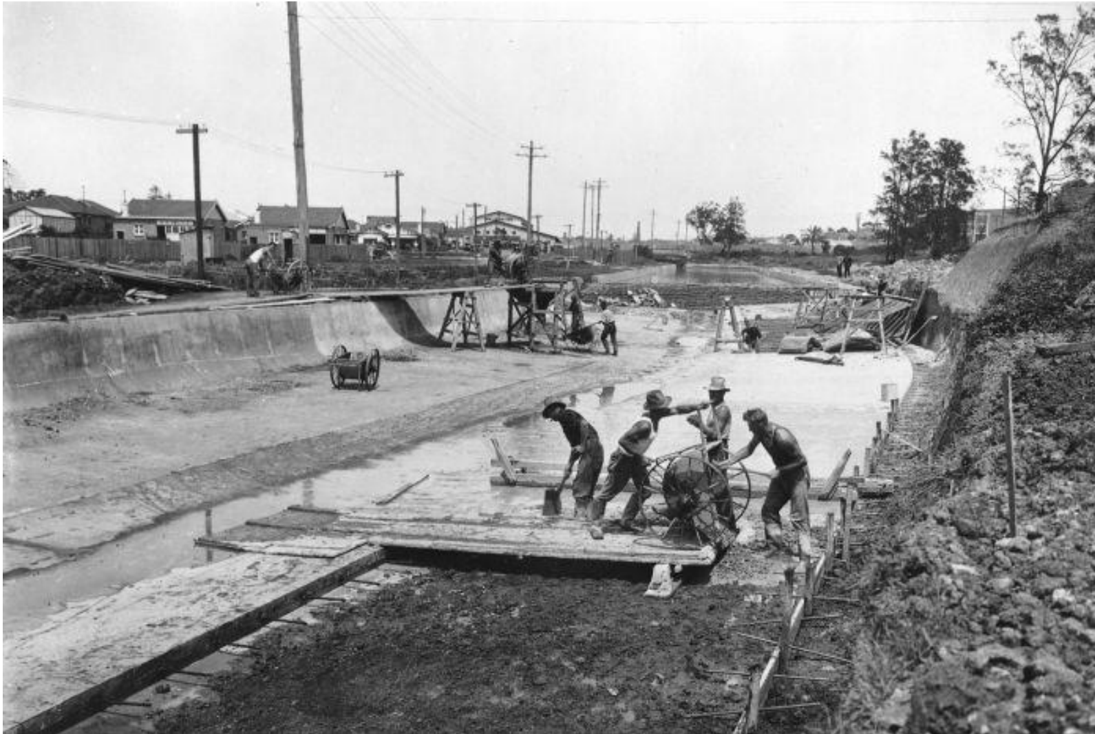
Figure 8. Construction of Hawthorne Canal at Haberfield, c.1926-1929 (Source: Sydney Water via ABC News, accessed online https://www.abc.net.au/news/2018-06-21/what-happened-to-sydneys-grand-plans-for-a-system-of-canals/9859904 )
