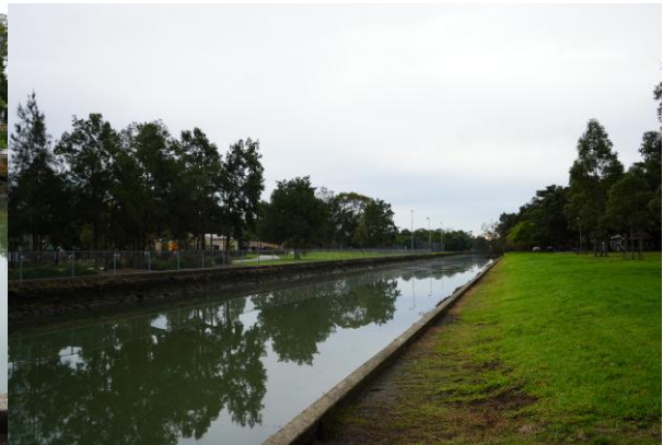
Figure 31: Looking northwest towards the canal retaining walls and Richard Murden Reserve, from western boundary of study area
