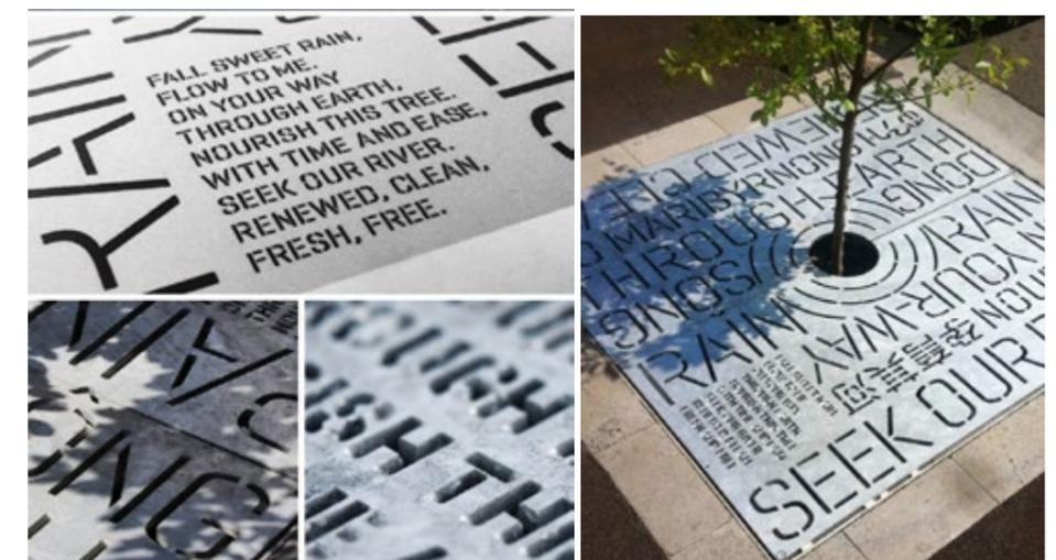
Figure 4.16 Examples of feature tree grate
