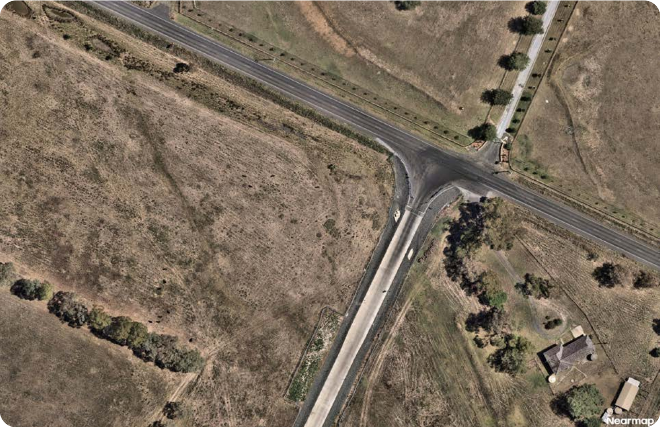
Above: Entrance into transformer substation along Calala Ln, NSW 2340.
