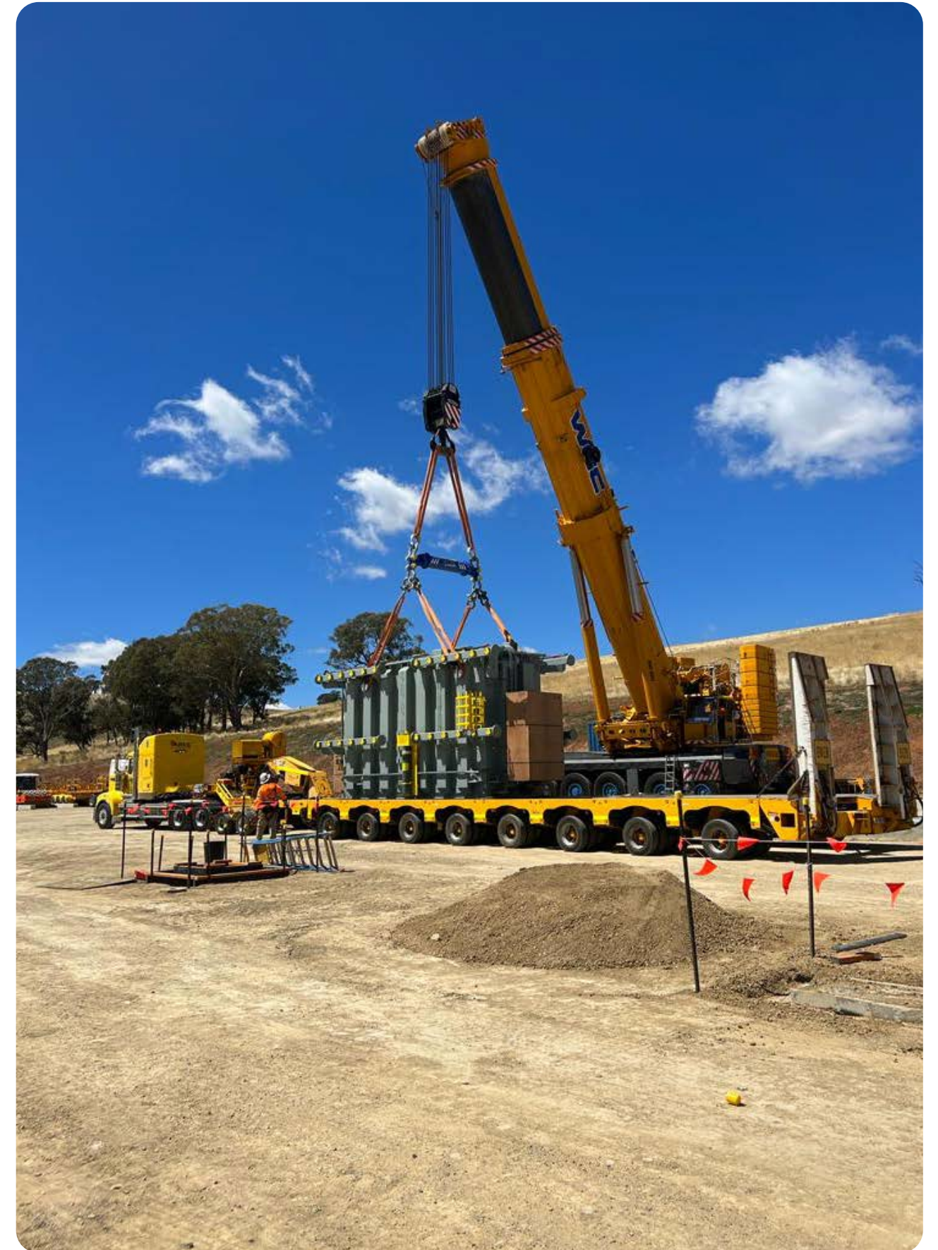
Above: ARES transporting a 120-ton transformer on a platform trailer to Flyers Creek Wind Farm.
