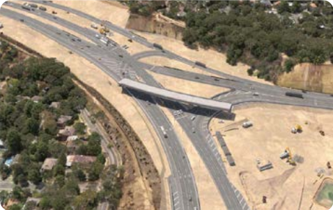
Above: North East Link - Greensborough Bypass to M80 Ring Road, interchange bridge pieces being constructed. (source: Victorias Big Build)
