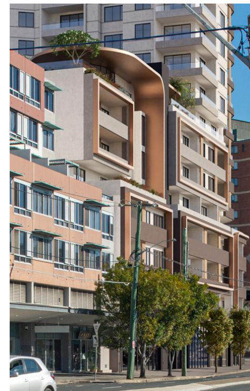
Figure 5: Extract of Forest Rd podium demonstrating copper 'fin' feature as well as various material depth (Source: Ivolve Studios)
