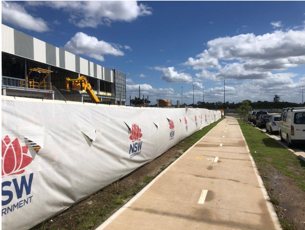
Figure 2-4 Shared path on Northbourne Drive, frontage to the school
