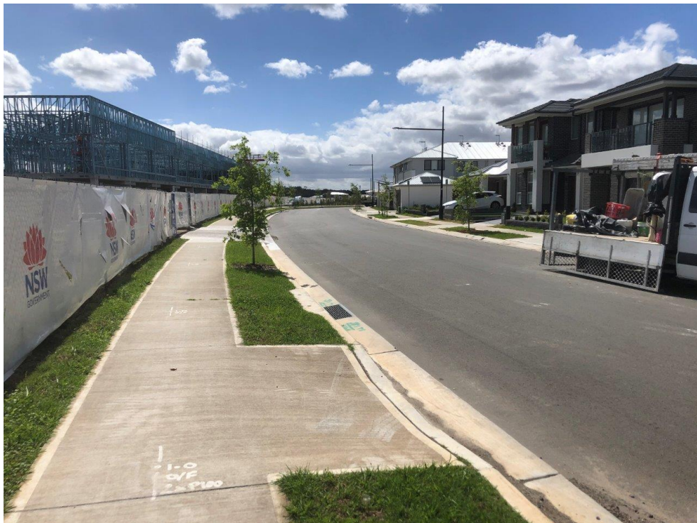
Figure 2-7 Pedestrian Footpaths on Enmore Street
