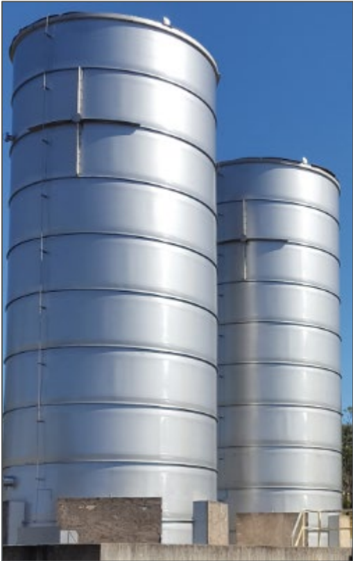
Plate 6: Vertical Flares (as used at permanent facilities)
