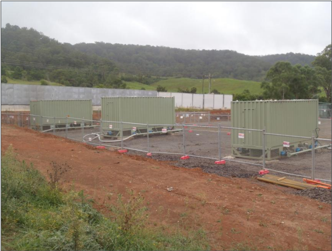
Plate 6: Vertical Flares (as used at permanent facilities)
