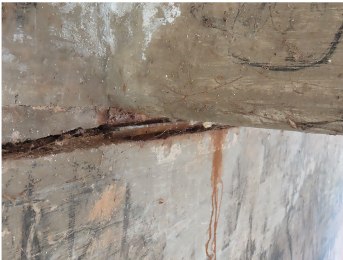
Photo 13. Tooma abutment (east end) bearing. Note on WAE drawings as a “fixed” abutment.
