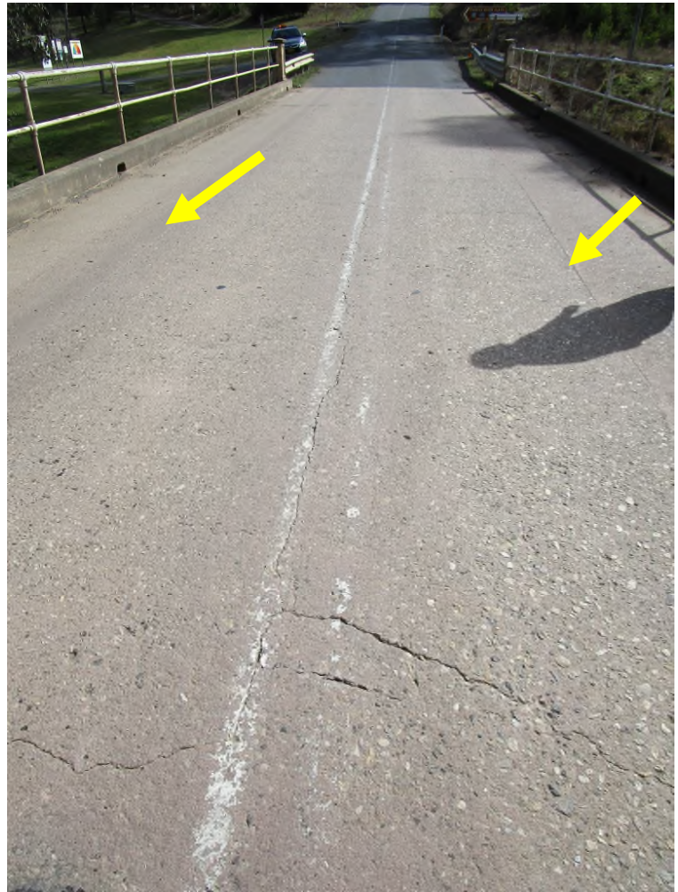
Photo 17. Transverse cracks in centre portion of deck. Note longitudinal construction joints (arrowed)
