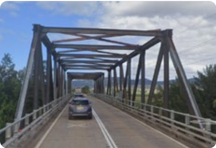
Above: Denman Bridge - 5.8m clearance.
