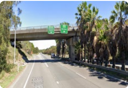
Below: Tarro Interchange overpass - 6.2m clearance.
