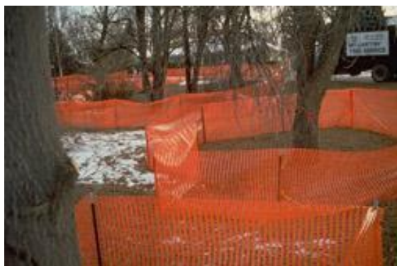
Figure 3. Example project Tree Protection Zone plastic barrier mesh fence
