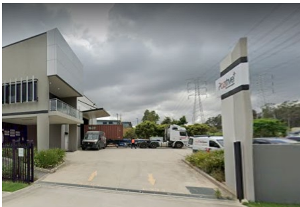
Figure 18: Buildings on the corner of Raceway Place proposed to be demolished on western boundary
