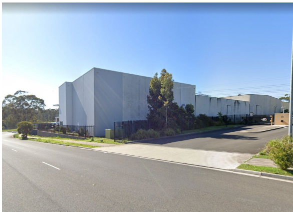
Figure 16: The existing Data Centre on Peter Brock Drive
