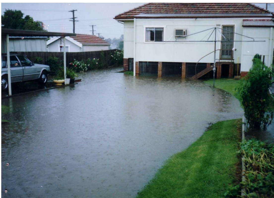
Floodwaters in rear yard of No. 22 Whitworth Street, Westmead during storm in 1990 (date unknown). [Domain Creek Catchment]
