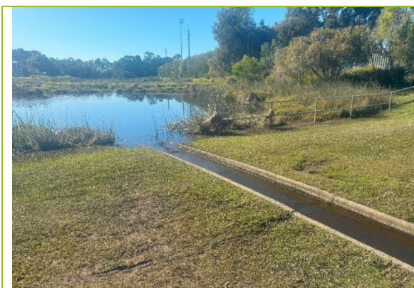
Photo 1: drainage channel and constructed wetland shown in area of potential 300mm increase during 1% AEI (viewed from south-southwest)
