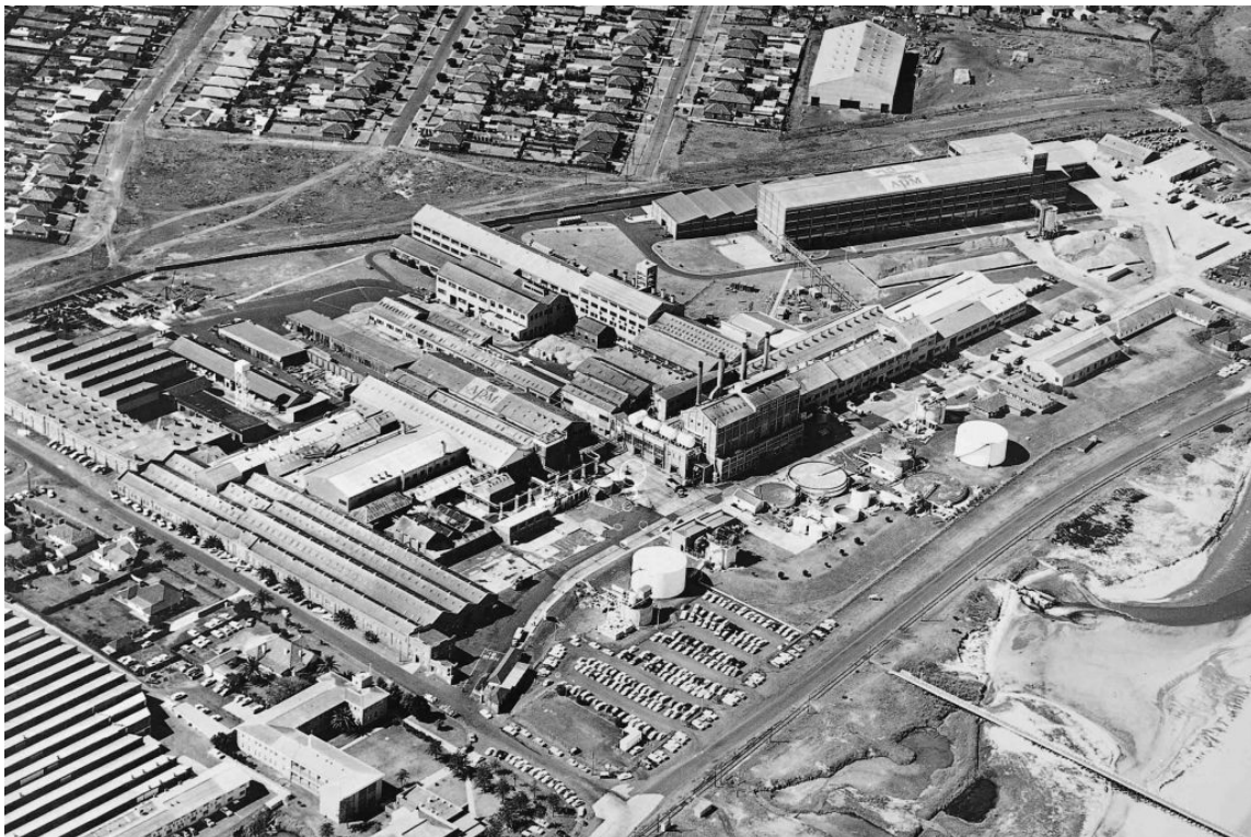
Plate 3.4: c.1970 aerial of Australian Paper Manufacturers, pier visible at far right. (Source: OPAL ANZ, 2026).
