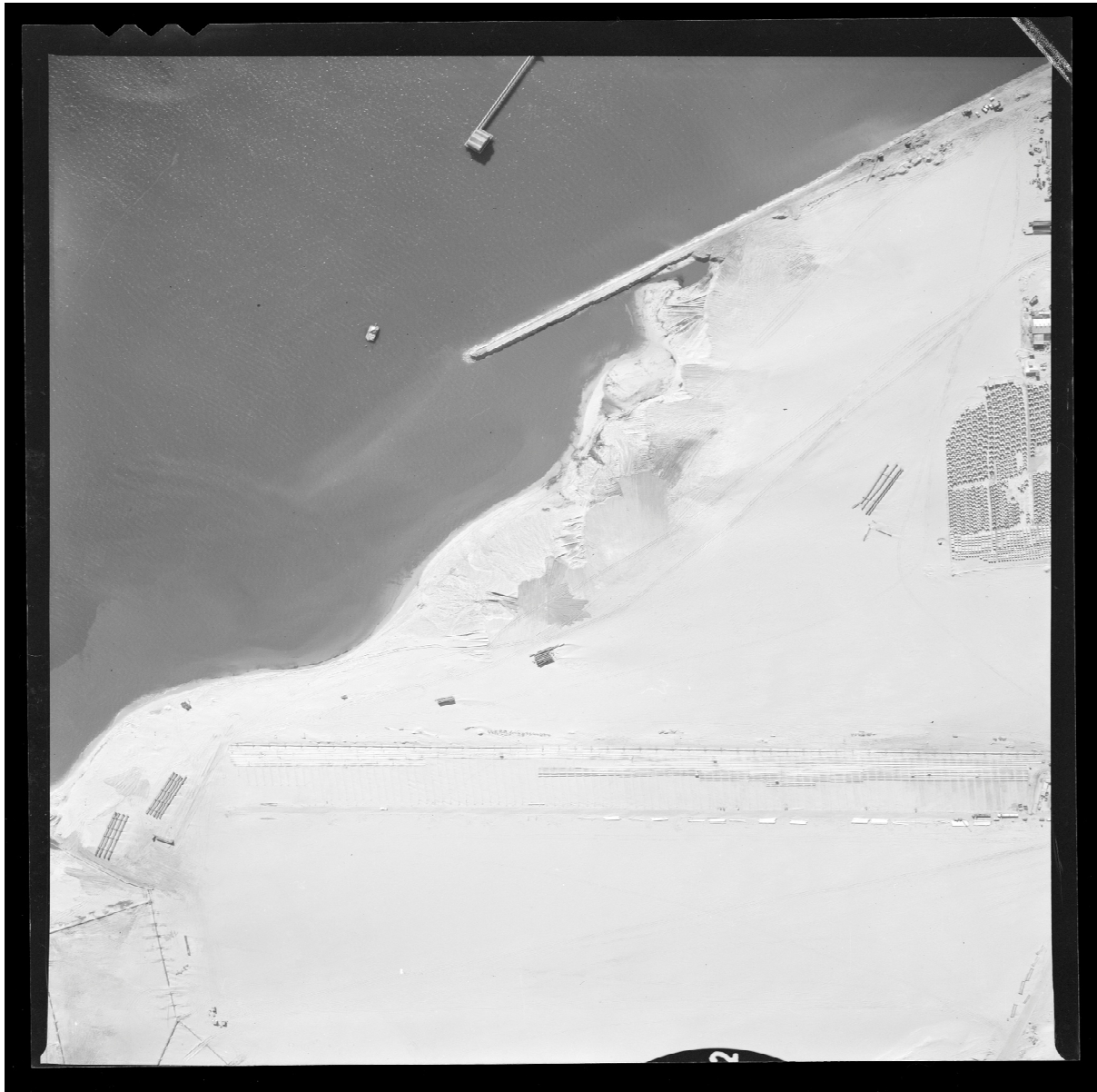
Plate 3.11: 1972 Milton Kent aerial showing construction of Brotherson Dock Two, north up, with APM pier top middle (Source: SLNSW, ON 447/Box 032).
