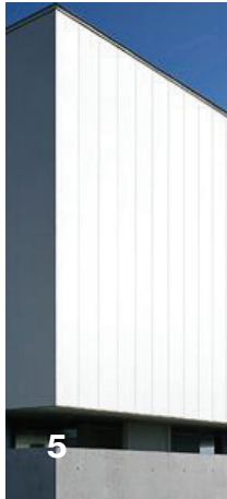
C. Metal Cladding
