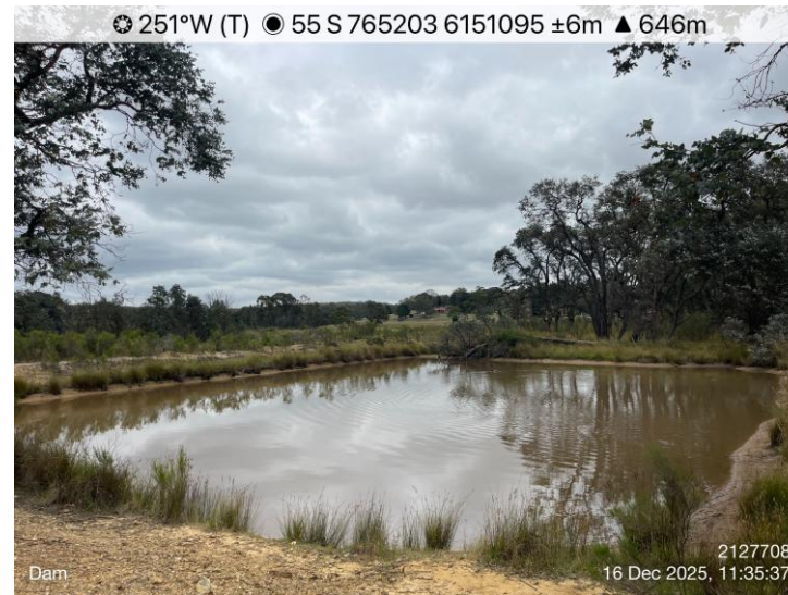
Photo 22: View looking west at the dam located in the south-west of the site (16/12/2025)
