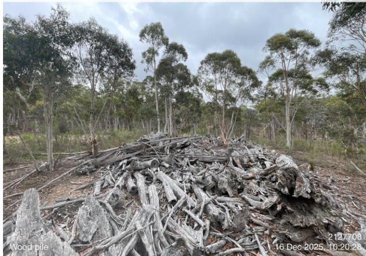
Photo 25: Example of wood stockpiles left over from the clearing for the internal gravel access road on Lot 3 (16/12/2025).
