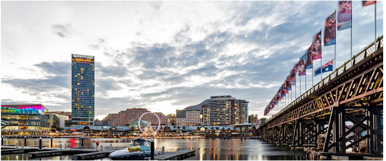
Existing Pyrmont Bridge
