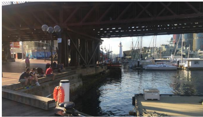
Existing Public Realm under Pyrmont Bridge
