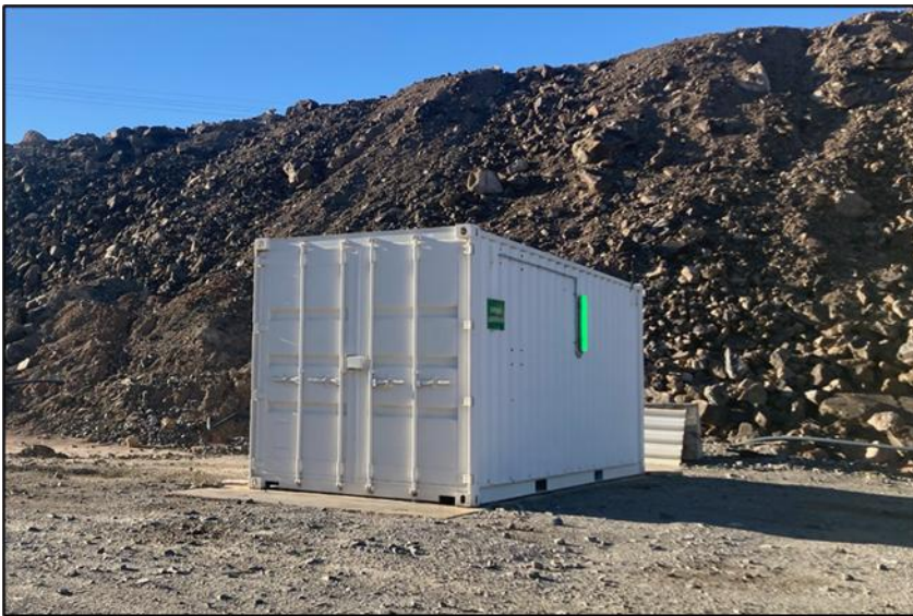
Figure 3: The Rasp Mine surface escape ladder way exit housing that was approved in MOD9.
