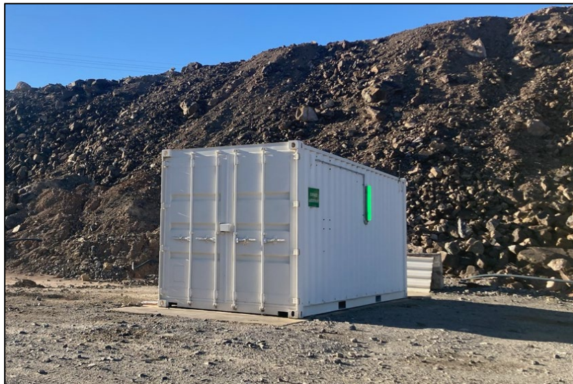
Figure 5: The Rasp Mine surface escape ladder way exit housing that was approved in MOD9.
