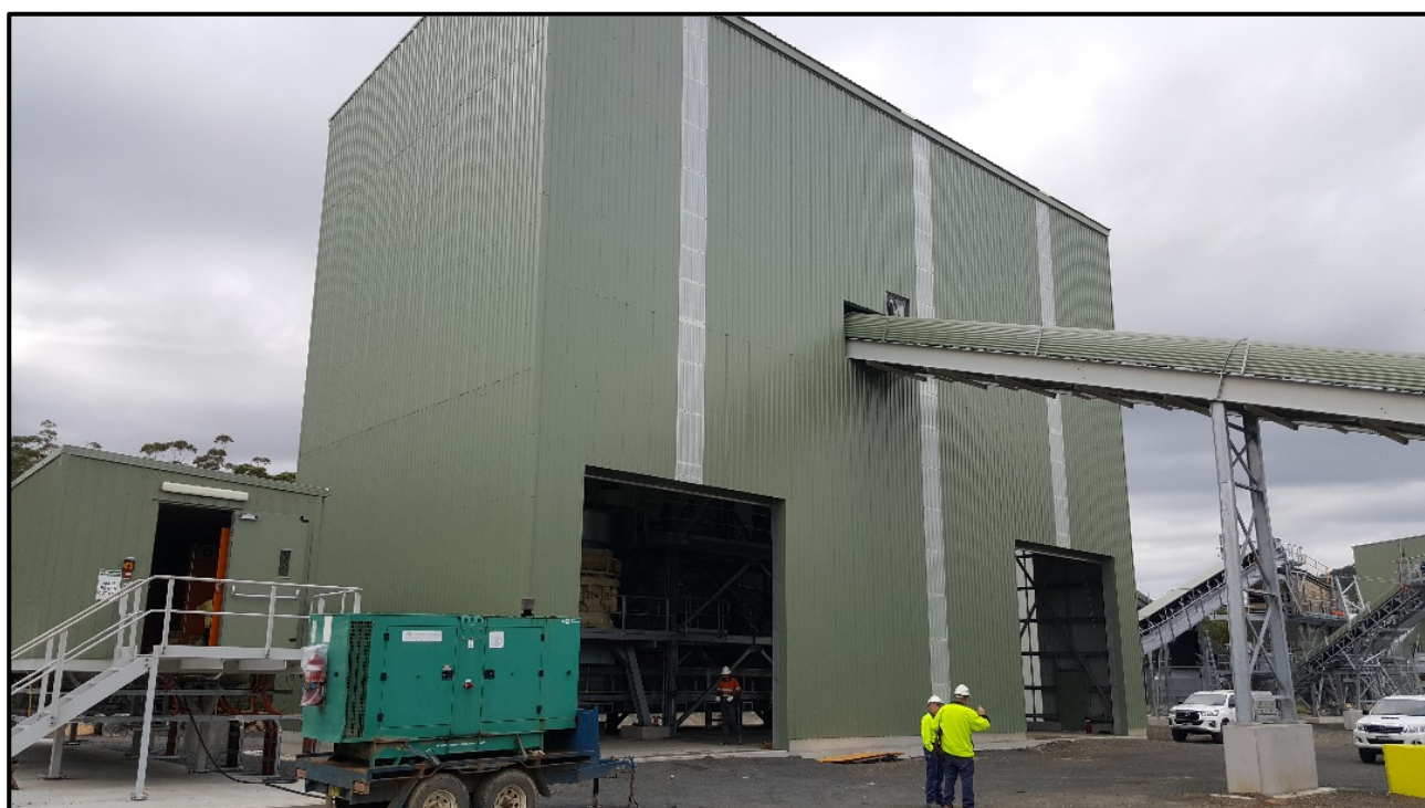
Figure 7: Secondary Cone Crusher Enclosure.
