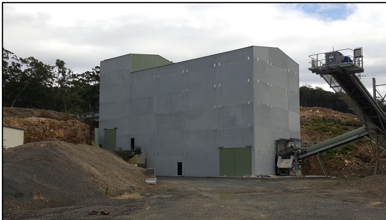
Figure 6: Primary Jaw Crusher Enclosure.
