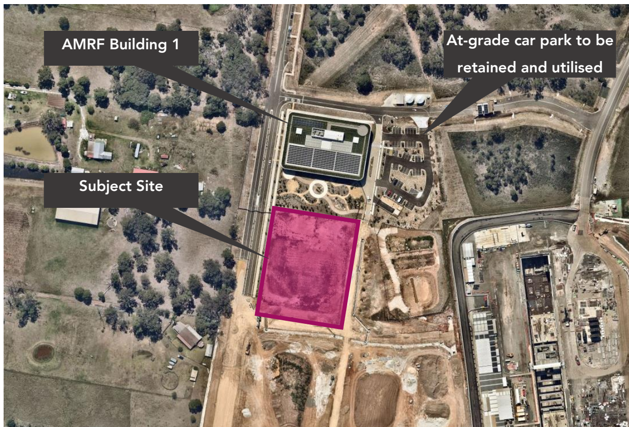
Figure 3 - The Site as at February 2025
