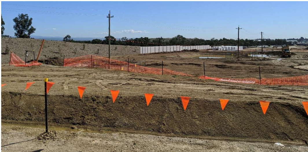
Figure 10: Bunding and noise wall currently under construction on western boundary (Source: Keylan)
