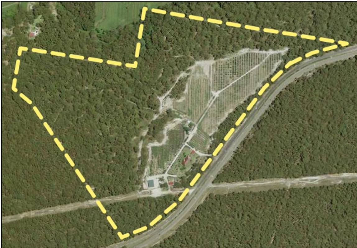
Figure 3: Local Context (aerial)
