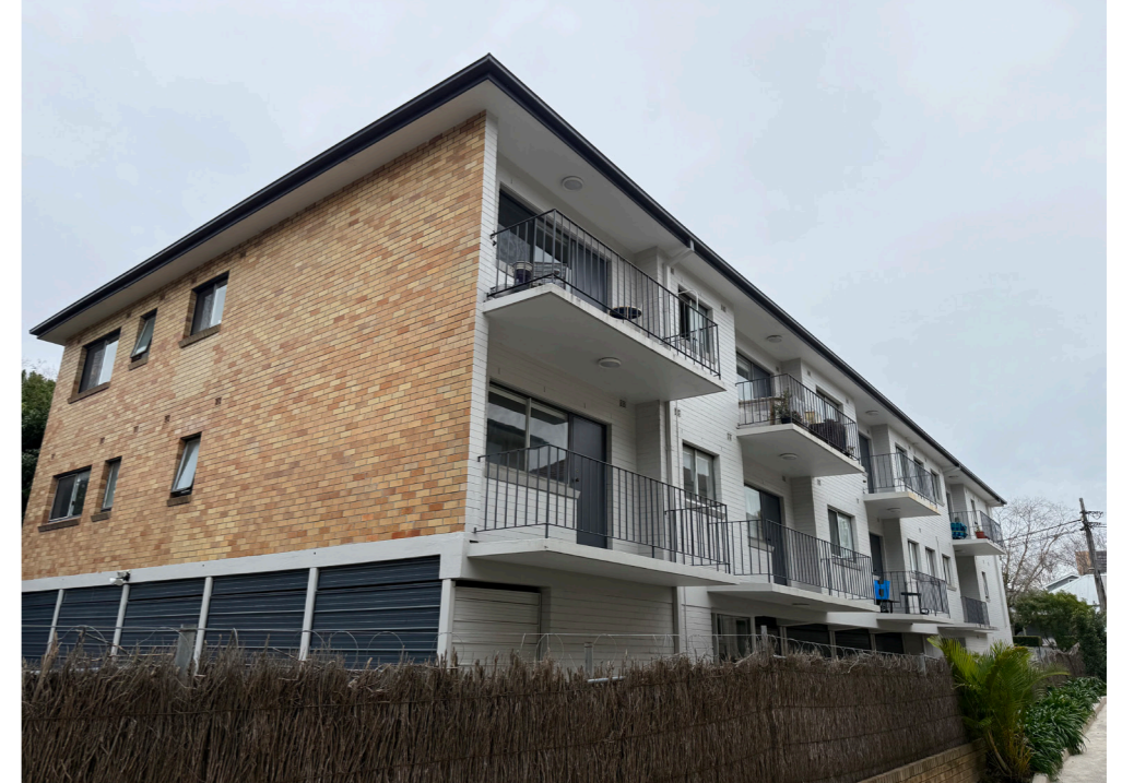
185-187 WEST ST Large carpark and small bedroom & bathroom windows facing our site, apartments face N/S
