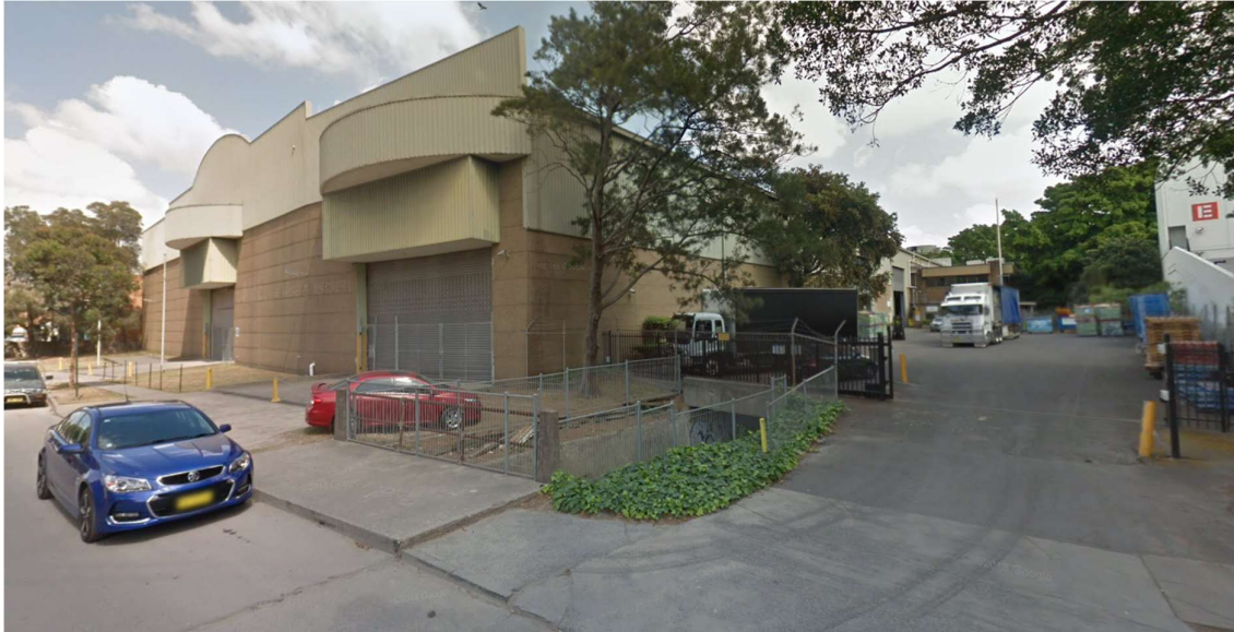
Figure 4. Street view of the site from Burrows Road showing the entrance to the main car park at right and the large existing building at left. The office building is at the far end of the car park and the stormwater culvert can be seen in the foreground.
