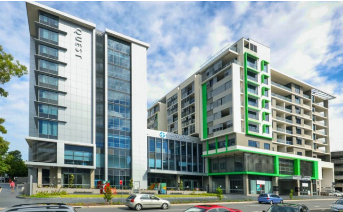
VIEW 01 View of the Quest Hotel from Albert Street
