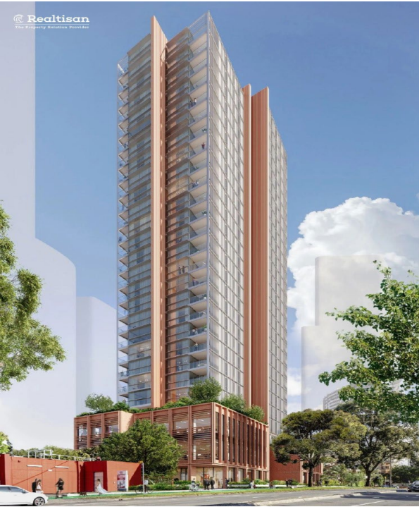
THE BRYSON 871-877 Pacific Highway
