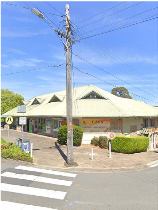
2. View of retail uses on Bank Street
