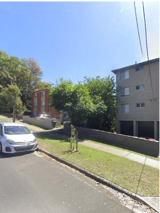
4. Residential buildings on Station street
