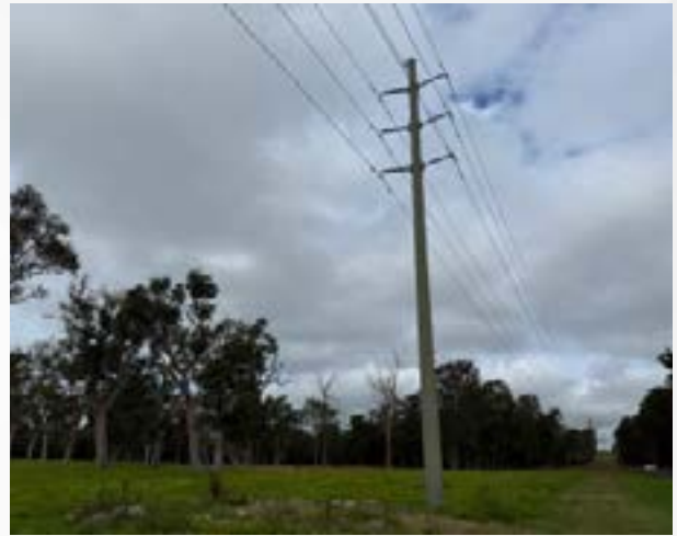
Photograph 4 x2 132kV transmission line looking south
