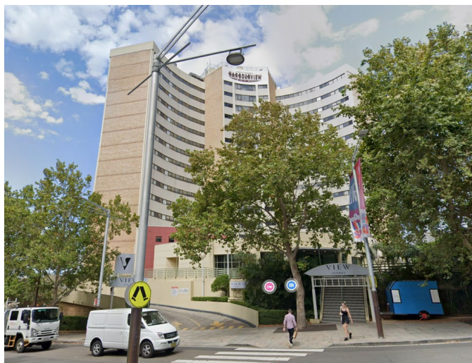
Figure 9 North-east of the site: View Sydney hotel
