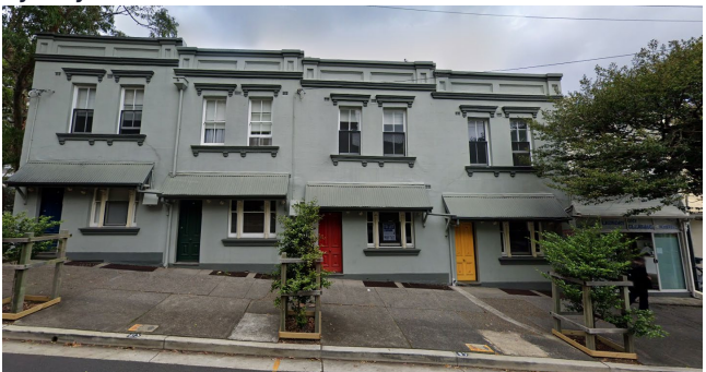
Figure 6 South-west of the site: Terraces
