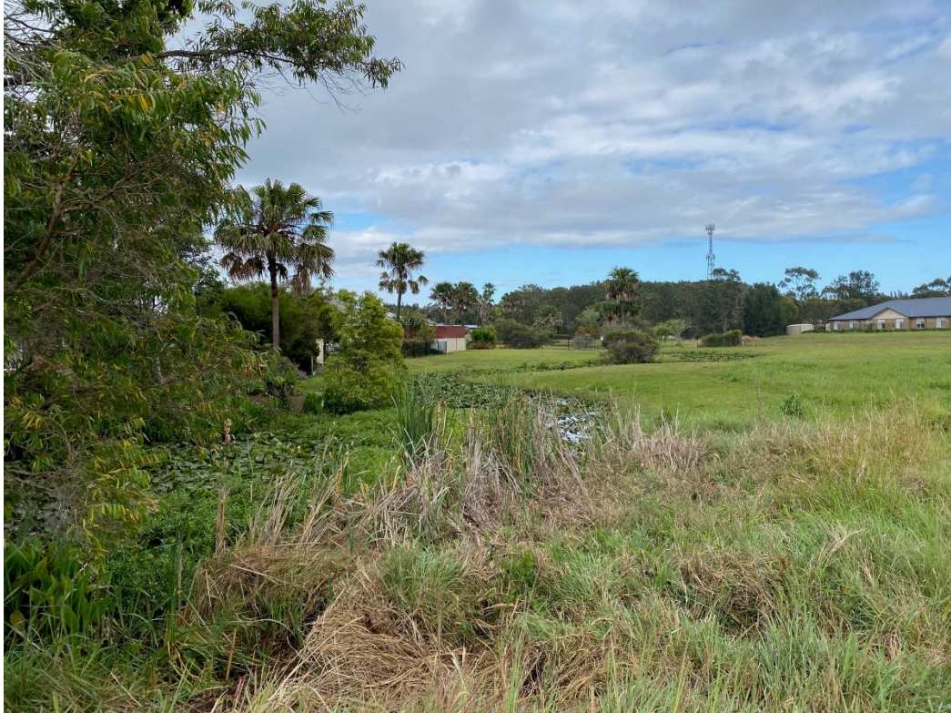
Existing stormwater drainage corridor
