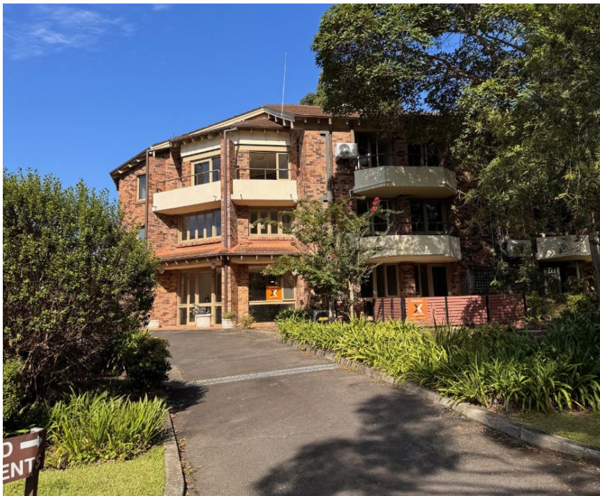
Figure 2 View of the site from the eastern entry from Stanhope Road
