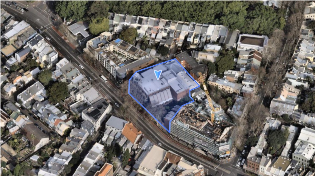
Figure 2 Aerial image of site context (looking south)
