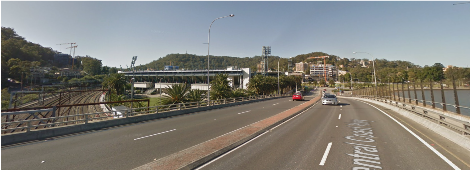
Existing view looking east from Gosford approach on Central Coast Highway
